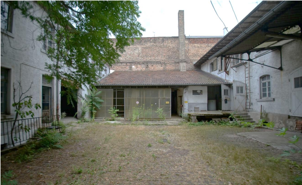
Figure 50: Connecting building between north- and south wing, Rudolfstrasse 5, Karlsruhe, Germany
