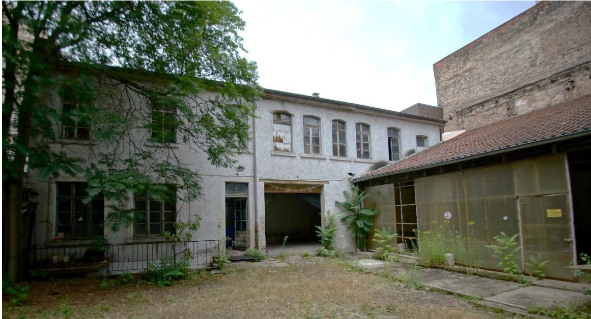
Figure 51: North wing of Rudolfstrasse 5, Karlsruhe, Germany
